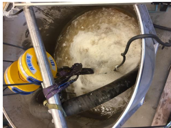
Fig. 2b: Pump submersed, Hose bent to recirculate flow
